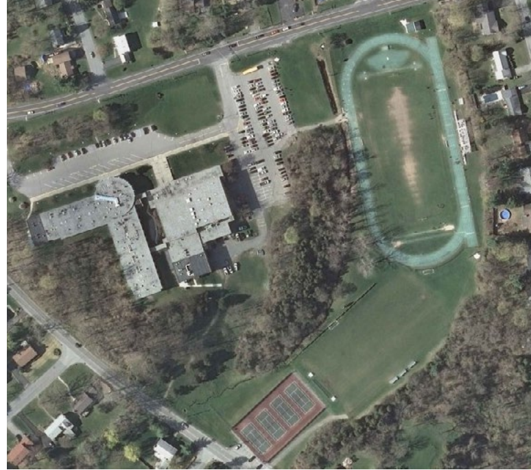
Figure 1: The state of the athletic fields at Spackenkill High School before the CIP, highlighting the need for urgent upgrades.
