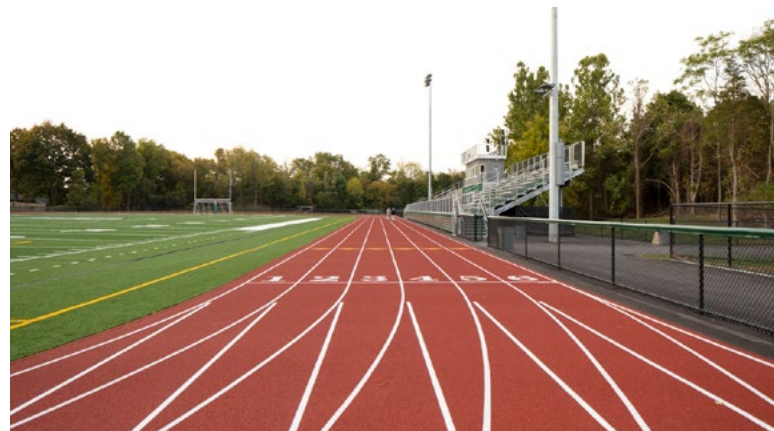
Figure 3: Spackenkill's repaved track.
