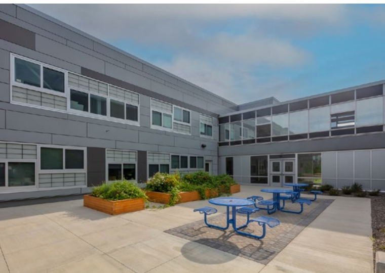
Figure 8 (above left) shows Monticello High's outdoor courtyard before the renovations. Figure 9 (left bottom) shows the updated courtyard, showing drastic improvements.
