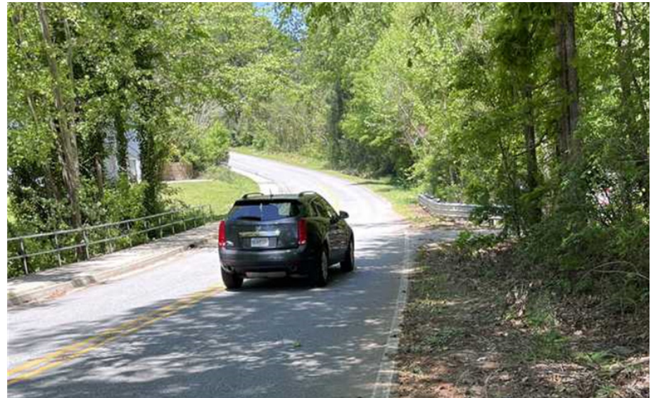
Figure 4 (H): Pedestrian Conditions at Alexander Avenue and Lakeside Drive
