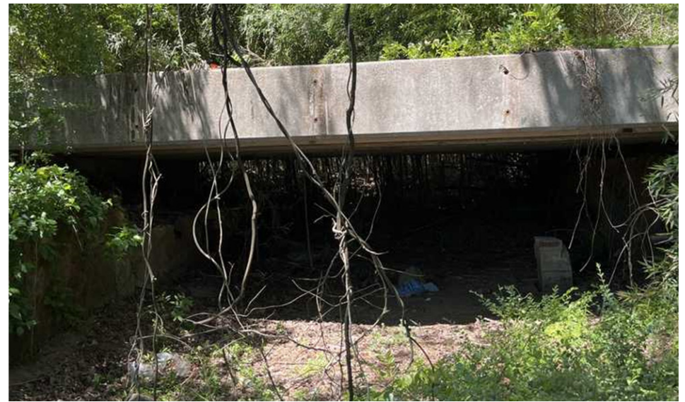
Figure 4 (D): Image of Concrete Bridge at Dixie Lake 2
